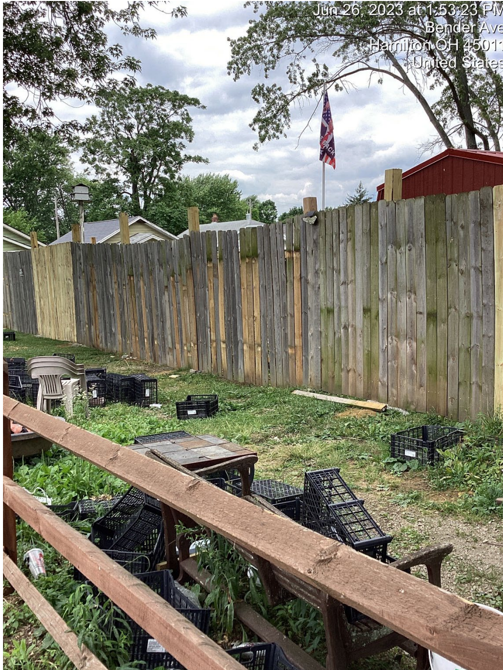
View of the fence along Bender Ave June 26
