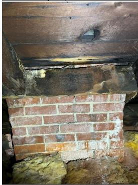
Interior Damage from Chimney Proposed to be Removed
