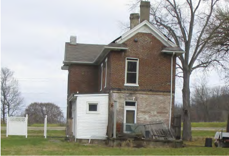
Photo of Rear of house- December 2016
