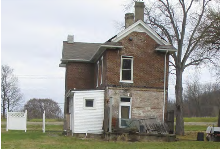
Photo of Rear of house- December 2016
